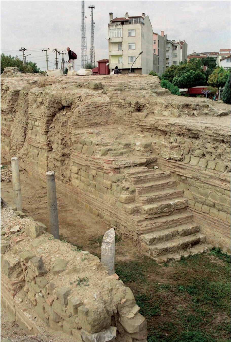
Plate 13. Herakleia Perinthos (Marmara Ereğlisi). Lower city walls next to the basilica.
